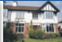
Turnberry, Prescot Road, Eccleston Hill
